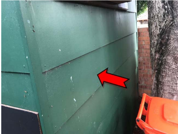
Photo 1. Exterior, throughout, wall paneling – non asbestos-containing fibre cement sheeting.
